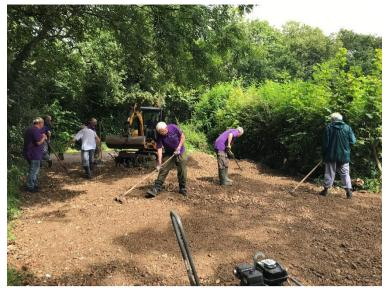
Two weeks later we moved onto Footpath 24. The bottom 2/3rds of this footpath were in a poor state, so again the same team moved Type 1 crushed limestone down the path to where it was being paid. This time though the path being narrower, the dumper had to be reversed all the way up! The final scrapings of the Type 1 were used to top up the head of the path to raise its level. This meant the surface was now higher than the remains of the stile, the stumps of which were trip hazards.
