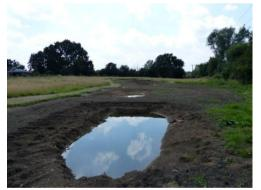
The excavations uncovered ancient field drainage pipes which if left untouched would have prevented the meadow becoming the wetland area we wanted. On the advice of experts Robert broke up the pipes and dug a trench between ponds and brook, backfilling with heavy clay effectively creating a barrier preventing drainage. This will mean the groundwater will rise and fill the ponds creating the wetland.
